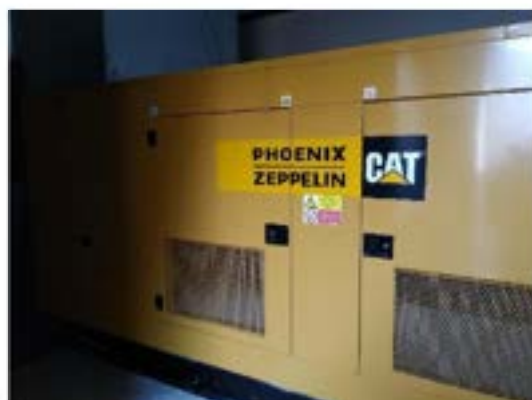
dieselagregát GEP450-4
