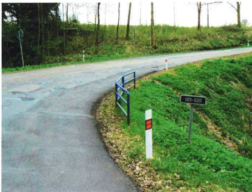
II/105, most ev.č. 105-020
