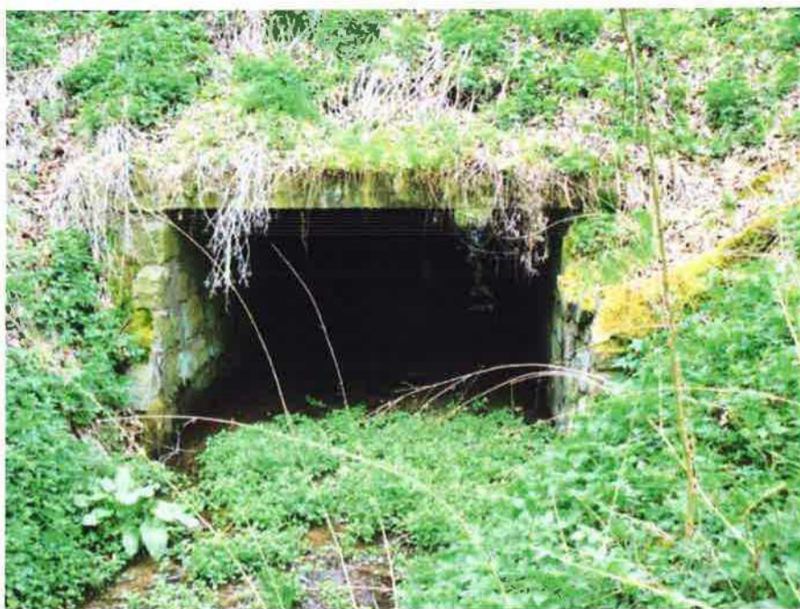
II/105, most ev.č. 105-020
