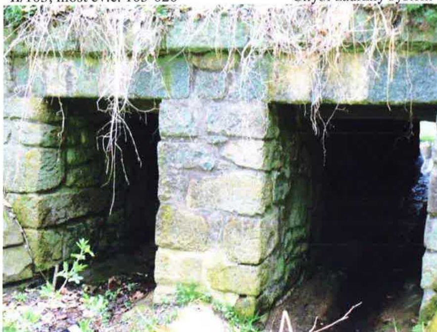
II/105, most ev.č. 105-020
