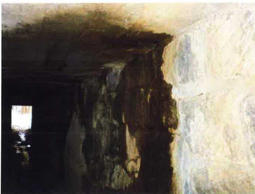
II/105, most ev.č. 105-020
