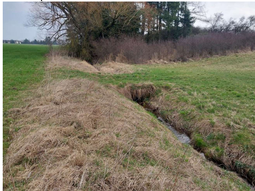
Propustek – naradit brodem
