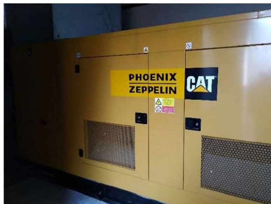
dieselagregát GEP450-4
