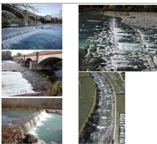
Left column: (top and middle) bed sills associated with a bridge; (bottom) bed sill Right column: (top) two bed sills connected by a boulder ramp, which impact on connectivity can be considered negligible; (bottom) a series of bed sills
