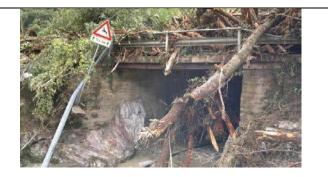
Bridge with a single arch of a low size High single arch bridge but with a small width, not enough to allow intense transport of large woods
