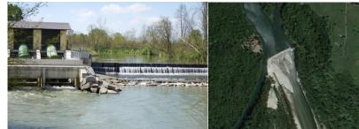
Top line: (left) abstraction weir with an abandoned mill; (centre) abstraction weir associated with an Archimedean screw hydropower plant; (right) Abstraction weir with movable gates.
