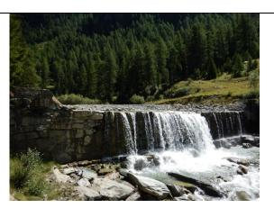
Consolidation weirs that are totally filled with sediments on the upstream side
