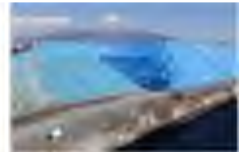
(Planar measures) Blue sheet coating
