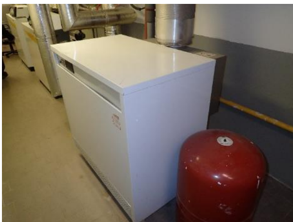
Obr. 194: Kotle Protherm a De Dietrich
