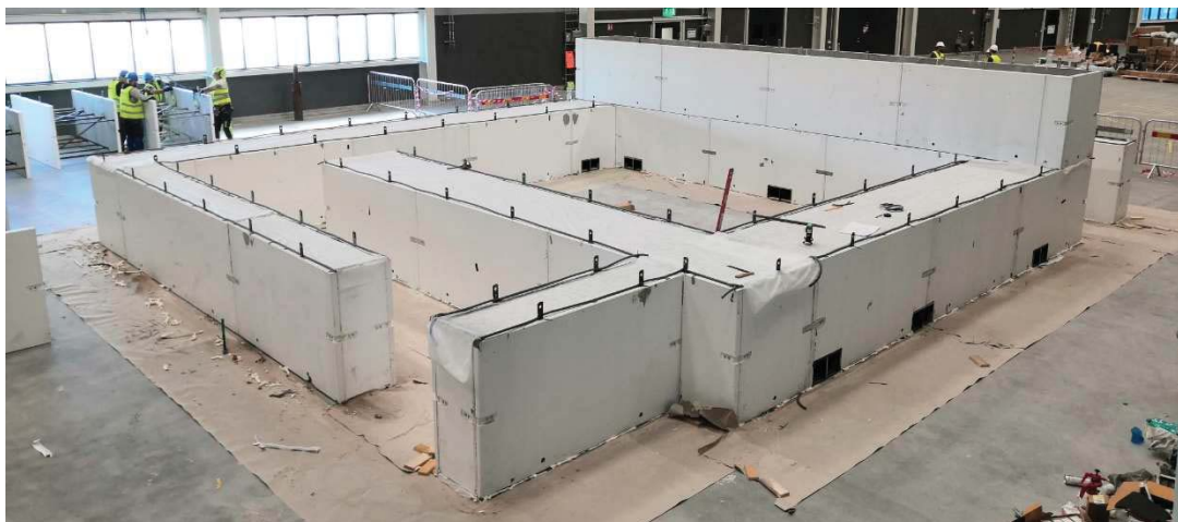
Fig. 7 – First layer finished, second layer assembled
