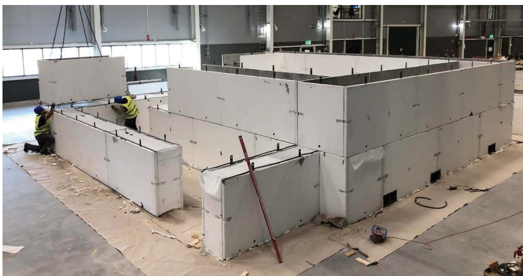
Fig. 8 – finishing second layer
