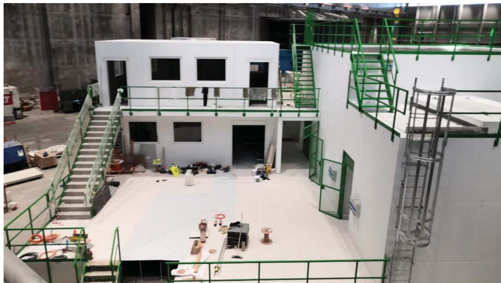
Fig. 11 – ESS DREAM cave and hutch under construction
