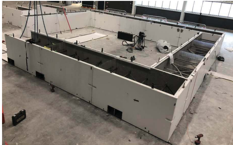
Fig. 5 – Partially assembled layer of segments, sep. Sheets inserted
