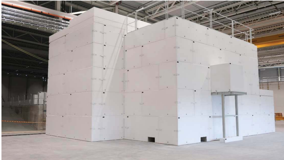
Fig. 10 – Finished ESS BIFROST cave structure (photo: Ulrika Hammarlund/ESS)
