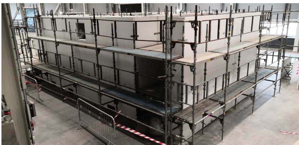
Fig. 9 – Third layer finished (state after just 13th day of installation Works)
