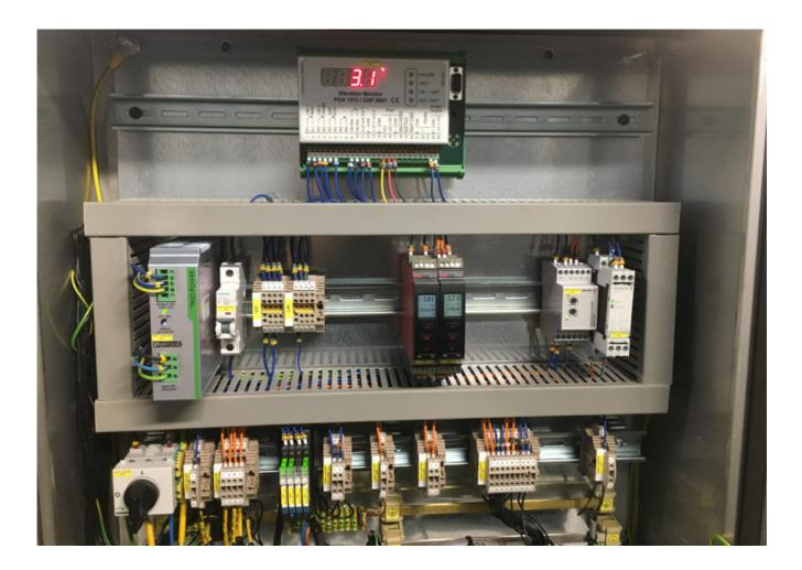
This shows a vibration of 3,1% = 31  $\mu$  peak-peak in empty running mode. The oil temperature shows 17,8°C.
