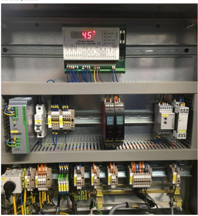
This shows a vibration of 4.5% =  $45~\mu$  peak-peak in empty mode running. The oil temperature shows 16.8 °C.
