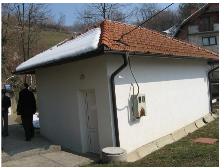
Figure 4: Capture of the source "Vrelo" and pumping station for Soko settlement
