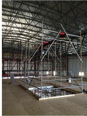
Figure 8b – Material Hoist
