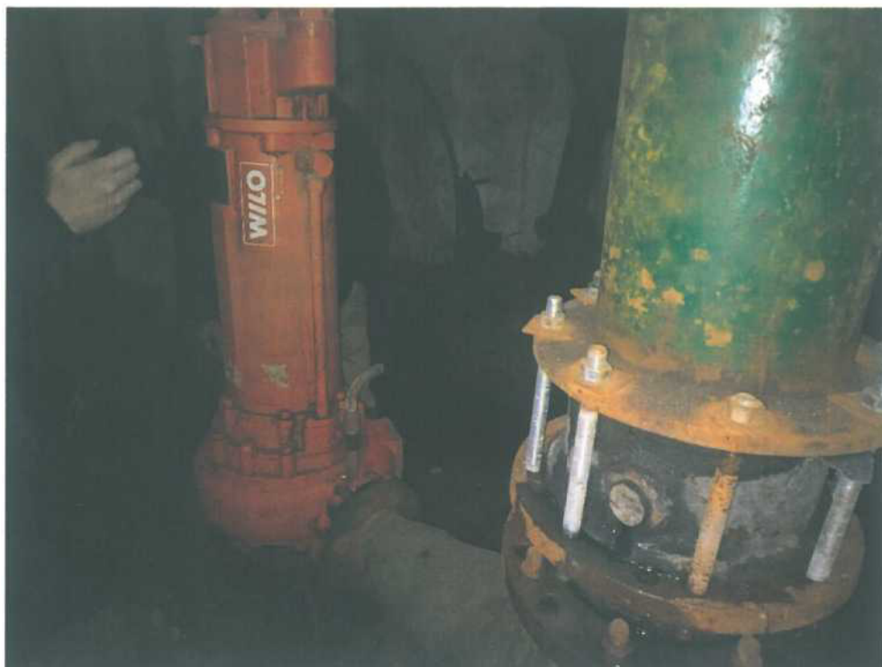
Fig. 8: View of the pumps in the main wastewater pumping station
