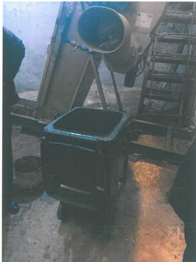
Fig. 7: View of the new mechanical pretreatment in the main wastewater pumping station, dustbin for scraps
