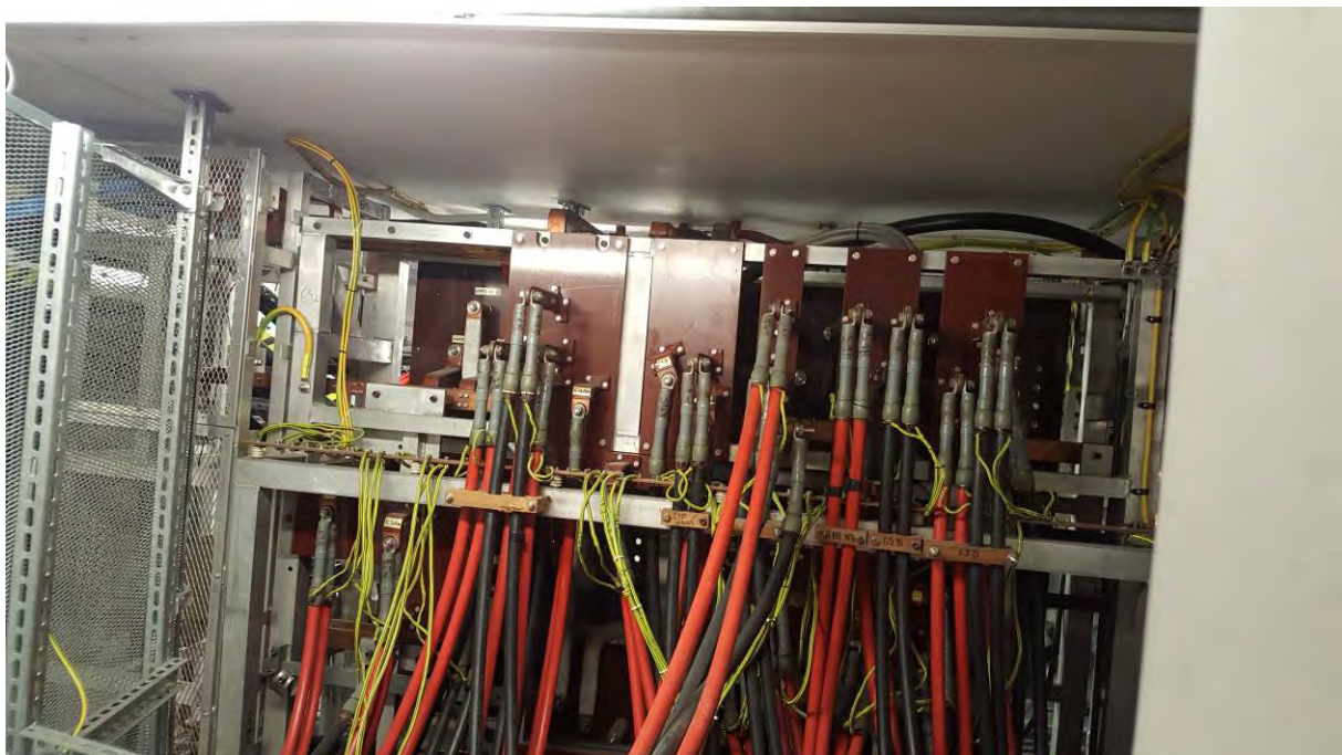
Figure 6.5.4: Picture of the connection point of the poloidal field coils
